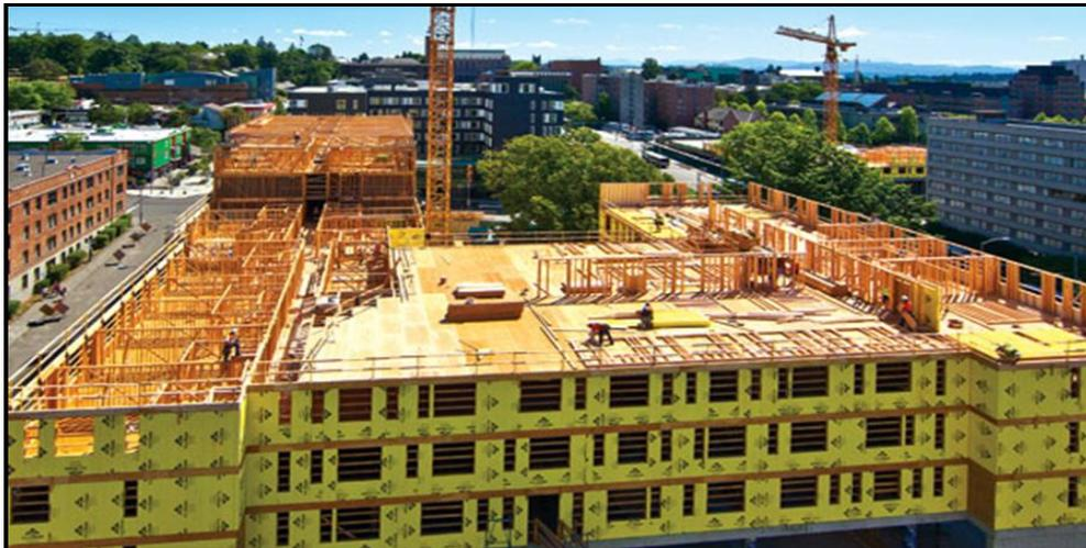
For this project in the Pacific Northwest, protecting wood from moisture was a priority. The yellow exterior sheathing is mold-resistant drywall. Although not shown in this photo measures to protect moisture ingress from rain, during construction, both from above and from wind-driven rain through the openings are equally important. Mold-resistant drywall is a 'post-construction' strategy.<sup>1</sup>
