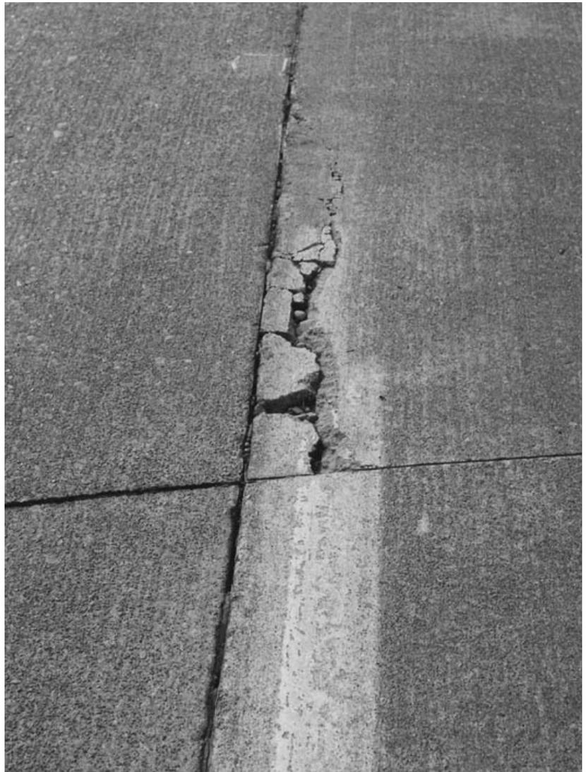
**Figure 11.** A typical location for a spall is along a joint, usually the result of the joint functioning improperly. (67216)
