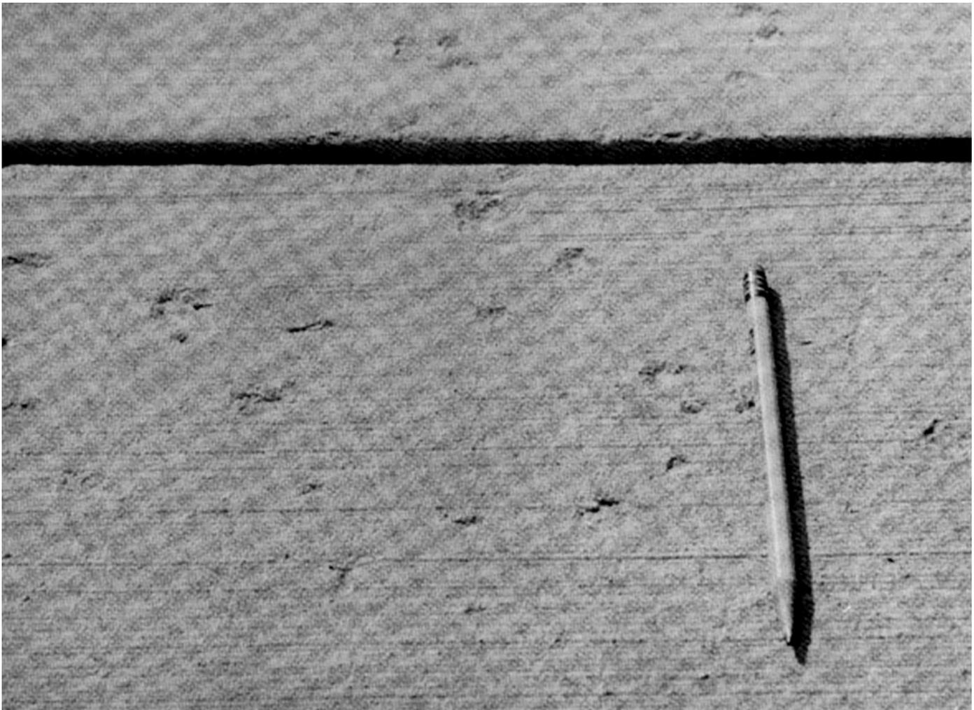
Figure 10. Mortar flaking over coarse aggregate. (52225)
