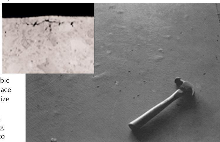
**Figure 1.** Blisters are surface bumps that may range in size from 5 mm to 100 mm (1/4 in. to 4 in.) in diameter with a depth of about 3 mm (1/8 in.). Inset photo cross section illustrates a void trapped under a blister. (Primary photo courtesy of National Ready Mixed Concrete Association.) (Inset, 49411; primary, A5272)
