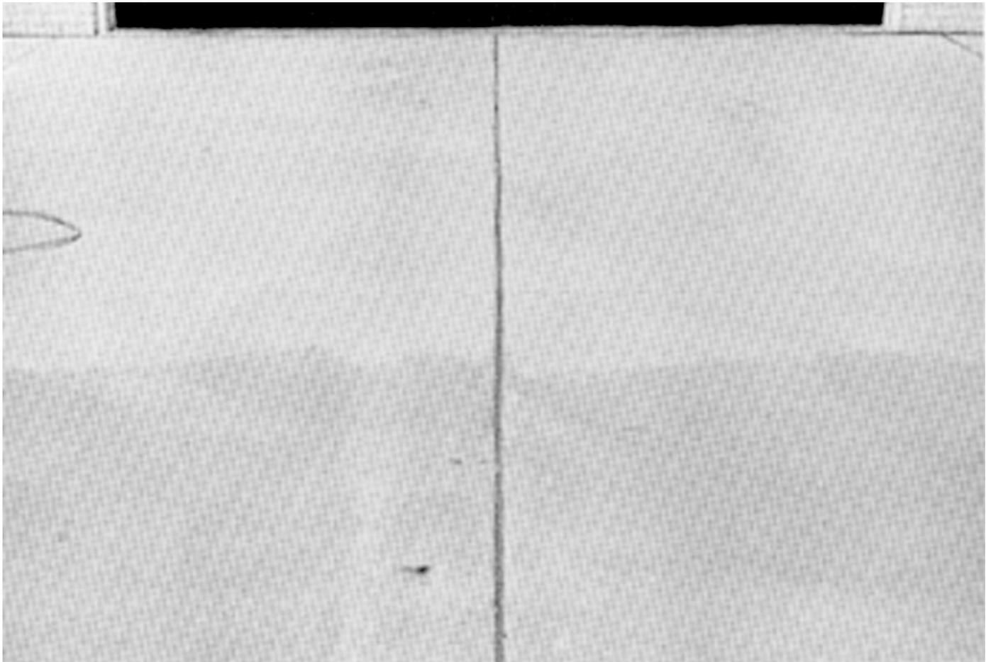
**Figure 6. Driveway discoloration due to the use of a calcium chloride admixture in the concrete at the bottom but not the top of the photo. This illustrates just one of several types of discoloration. (14019)**
