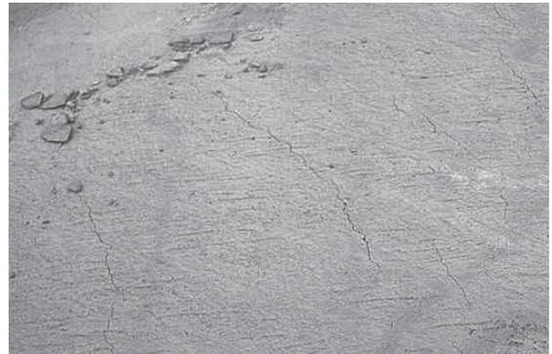
paste shrinks during early hydration which produces very small micro cracks. When the rate of evaporation is high and the concrete has enough strength (or stiffness) to cause horizontal shrinkage the normal micro cracking tendency is accentuated and noticeable plastic cracking may result.
