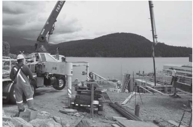
slides down the pipe, it develops a vacuum which greatly expands the air bubbles; and when they hit an elbow in the boom or a horizontal surface, the bubbles collapse. Naturally, the transition from several hundred MPa of pressure in the line to a near vacuum condition may make matters worse. Most field experience suggests that air loss is greatest with rich, flowable mixes which slide down easier; however, air loss has also been experienced with 300kg/m<sup>3</sup>.
