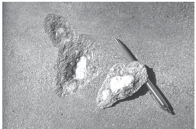
A popout is a small fragment of concrete surface that broke away due to internal pressure, leaving a shallow, typically conical, depression.
